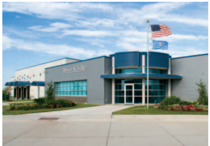
Bio-Cide International, Inc. the worldwide leader in Chlorine Dioxide technology.
