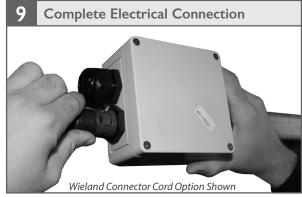
• Connect power cord from fixture to power supply.
