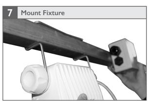
· Raise fixture to ceiling and slide mounting bracket over the track/truss; ensuring fixture is securely in place.
